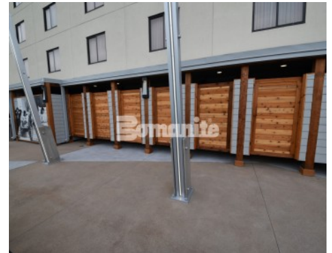
Hard Rock Hotel and Casino Tulsa Pool Deck - Bomanite Alloy Exposed Aggregate System
