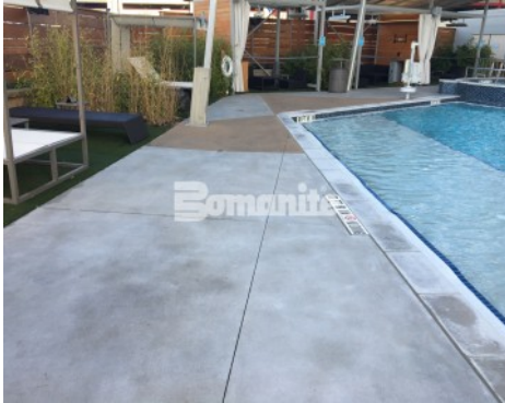
Hard Rock Hotel and Casino Tulsa Pool Deck - Bomanite Alloy Exposed Aggregate System
