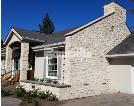
California Private Residence - Bomanite Imprint Systems English Sidewalk Slate Pattern Concrete Driveway
