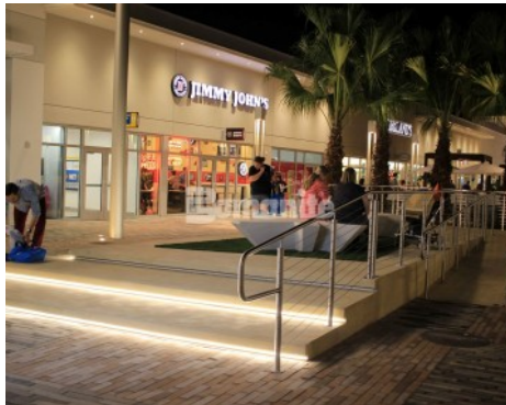
Tanger Outlets Daytona Beach - Bomanite Exposed Aggregate with Seashells Steps and Handicap Ramp
