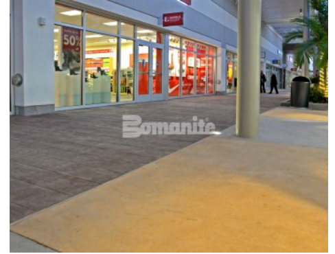
Tanger Outlets Daytona Beach - Bomanite Imprint Systems Bomacron Boardwalk Pattern Used in Store Front Walkway
