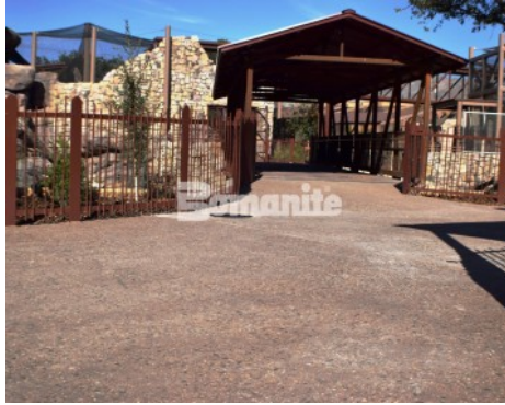
El Paso Zoo Chihauhaun Desert Exhibit - Bomanite Imprint 6" Boardwalk Pattern with Natural Exposed Aggregate
