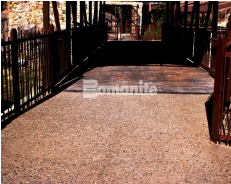
El Paso Zoo Chihuahuau Desert Exhibit - Bomanite Imprint 6" Boardwalk Pattern with Natural Exposed Aggregate
