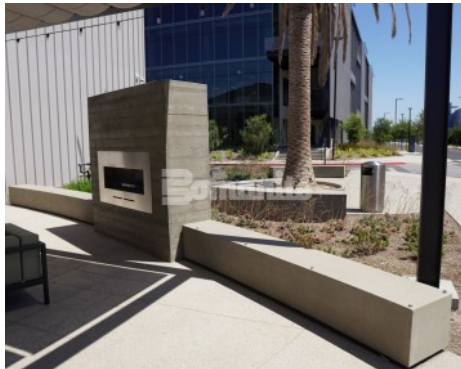
Flight at Tustin Legacy Business Development Campus - Bomanite Exposed Aggregate Revealed Walkway and Seat Wall, Board Formed Fire Hearth
