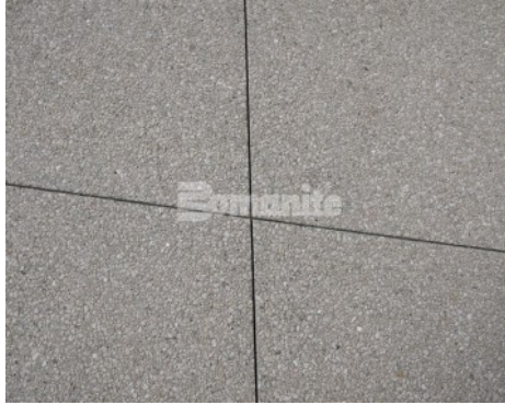
Flight at Tustin Legacy Business Development Campus - Bomanite Exposed Aggregate Revealed Walkway Close Up
