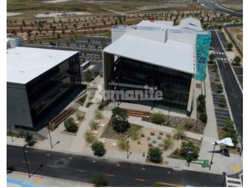
Flight at Tustin Legacy Business Development Campus - Bomanite Exposed Aggregate Revealed Courtyard
