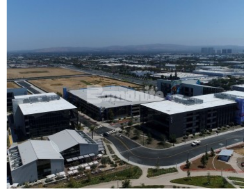
Flight at Tustin Legacy Business Development Campus - Bomanite Exposed Aggregate Revealed
