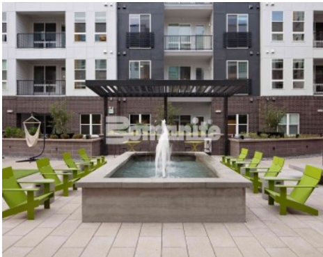
CoLab Community Housing - Bomanite Exposed Aggregate Sandstone Texture Walkways with Board-Formed Concrete Water Feature
