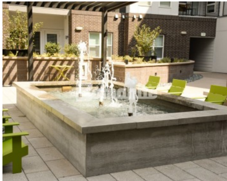
CoLab Community Housing - Bomanite Exposed Aggregate Sandstone Texture Walkways with Board-Formed Concrete Water Feature
