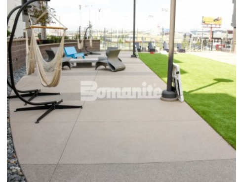
CoLab Community Housing - Bomanite Exposed Aggregate Sandstone Texture Walkways in alternating colors
