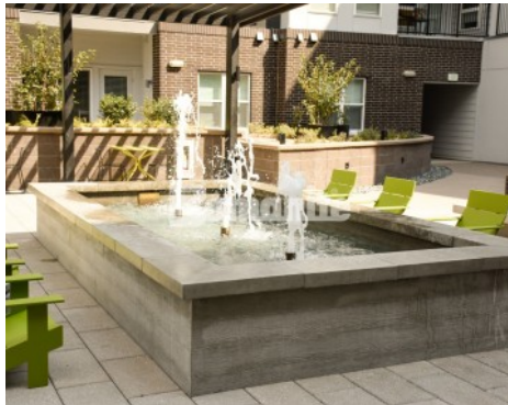
CoLab Community Housing - Bomanite Exposed Aggregate Sandstone Texture Walkways with Board-Formed Concrete Water Feature
