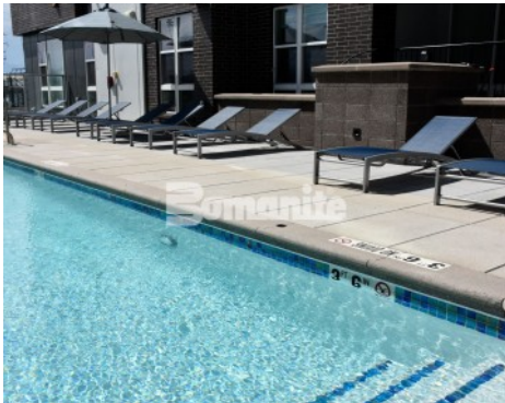
CoLab Community Housing - Bomanite Exposed Aggregate Sandstone Texture Pool Coping
