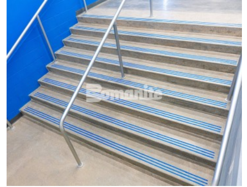
Grain Valley High School Renovation - Bomanite Custom Polishing Modena SL with Epoxy filled stair treads
