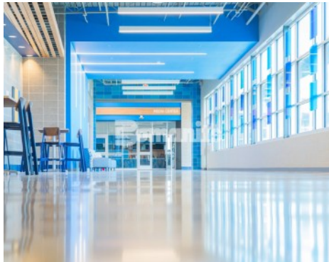
Grain Valley High School Renovation - Bomanite Custom Polishing Modena SL Interior Hallway with Cream Polish Salt and Pepper Aggregates
