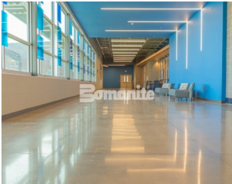
Grain Valley High School Renovation - Bomanite Custom Polishing Modena SL Interior Hallway with Cream Polish Salt and Pepper Aggregates
