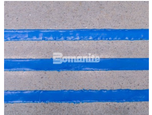
Grain Valley High School - Bomanite Custom Polishing Modena SL with Epoxy filled stair treads
