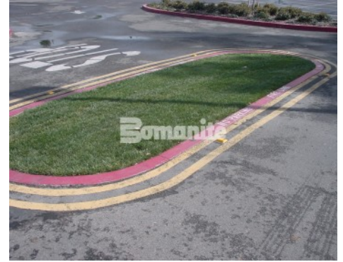
Woodbury Community Development - Grasscrete Emergency Vehicle Access Median
