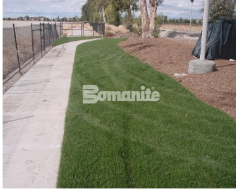
Woodbury Community Development - Grasscrete Emergency Vehicle Access Jeffrey Trail
