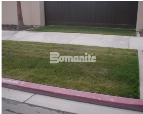
Woodbury Community Development - Grasscrete Emergency Vehicle Residential Access
