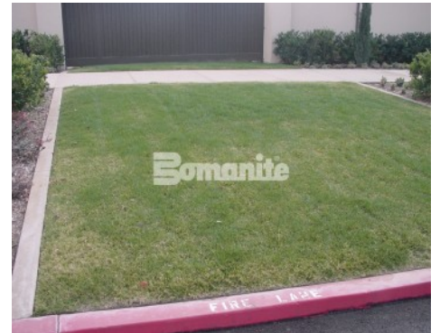
Woodbury Community Development - Grasscrete Emergency Vehicle Residential Access
