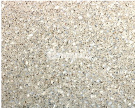
MMGY Global Marketing Firm - Bomanite Modena SL Polished Concrete Floor Close Up
