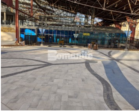
St. Louis Aquarium at Union Station - Bomanite Revealed Exposed Aggregate River Confluence Entry
