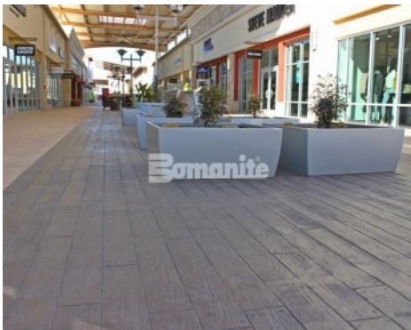
Target Outlets Fort Worth - Bomanite Imprint Systems Walkways - Boardwalk Pattern
