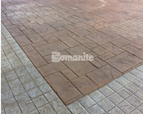
Target Outlets Fort Worth - Bomanite Imprint Systems Walkways - 6" x 6" Granite Setts, Medium Ashlar Slate
