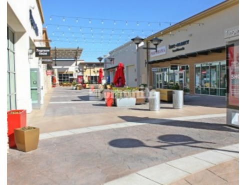
Target Outlets Fort Worth - Bomanite Imprint Systems Walkways - Canyon Stone, Used Brick Texture, Medium Ashlar Slate
