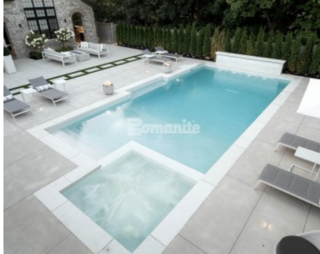
Kleinburg Residential Patio and Pool Deck - Bomanite Sandscape Refined Exposed Aggregate System
