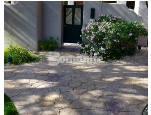
Villas of Cave Creek - Bomanite Imprint Systems - Canyon Stone Pattern Walkways
