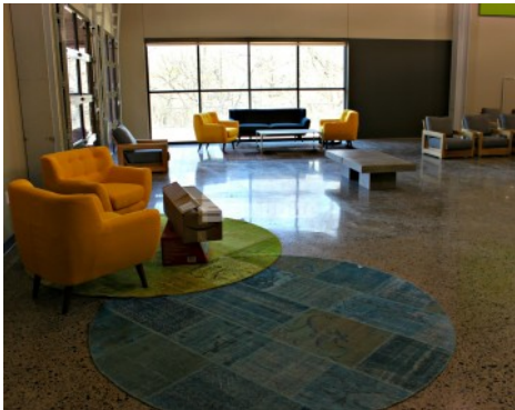
Chase Oaks Church Fairview TX - Bomanite VitraFlor Polished Concrete with Black Aggregates
