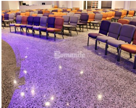
Chase Oaks Church Fairview TX - Bomanite VitraFlor Polished Concrete with Black Aggregates
