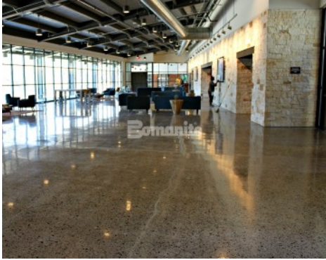
Chase Oaks Church Fairview TX - Bomanite VitraFlor Polished Concrete with Black Aggregates
