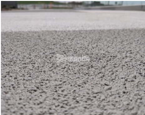
Cerner Campus Entrance - Bomanite Micro-Top XT and Bomanite Micro-Top ST
