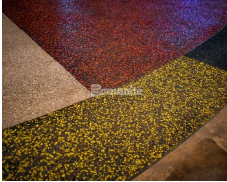
Choctaw Cultural Center - Bomanite Revealed Glass Aggregates in White, Black, Red and Yellow
