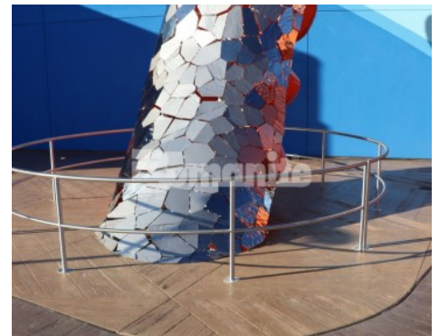
Branson Boardwalk Aquarium - Bomanite Imprint Systems Custom Hexagon Boardwalk Pattern with Custom 8' Radius Boardwalk Planks
