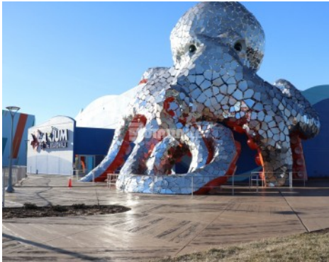
Branson Boardwalk Aquarium - Bomanite Imprint Systems Custom Hexagon Boardwalk Pattern with Custom 8' Radius Boardwalk Planks
