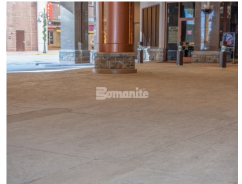
Monarch Casino Black Hawk Port Cochere - Bomanite Imprint Systems English Sidewalk Slate Texture with Bomanite Sandscape Texture Banding
