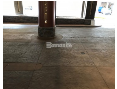
Monarch Casino Black Hawk Port Cochere - Bomanite Imprint Systems English Sidewalk Slate Texture with Bomanite Sandscape Texture Banding
