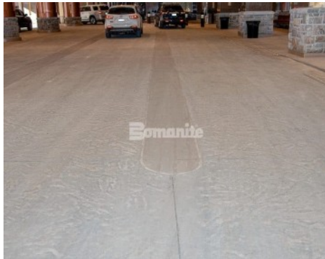
Monarch Casino Black Hawk Port Cochere - Bomanite Imprint Systems English Sidewalk Slate Texture with Bomanite Sandscape Texture Banding
