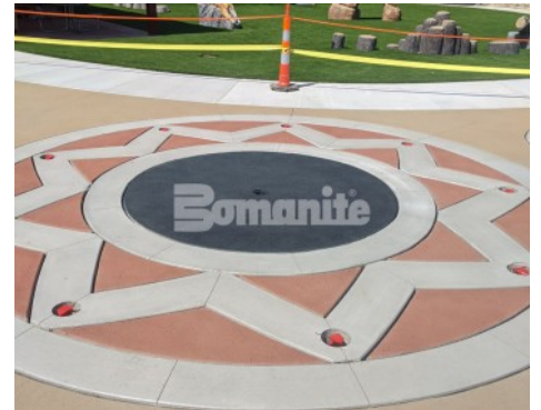
Community Park Jefferson City Splash Pad- Bomanite Sandscape Texture Exposed Aggregate with Bomanite Con-Color
