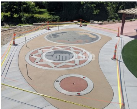
Community Park Jefferson City Splash Pad- Bomanite Sandscape Texture Exposed Aggregate with Bomanite Con-Color
