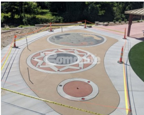
Community Park Jefferson City Splash Pad- Bomanite Sandscape Texture Exposed Aggregate with Bomanite Con-Color
