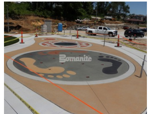
Community Park Jefferson City Splash Pad- Bomanite Sandscape Texture Exposed Aggregate with Bomanite Con-Color
