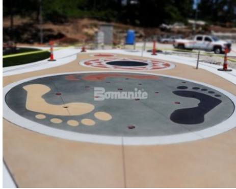
Community Park Jefferson City Splash Pad- Bomanite Sandscape Texture Exposed Aggregate with Bomanite Con-Color
