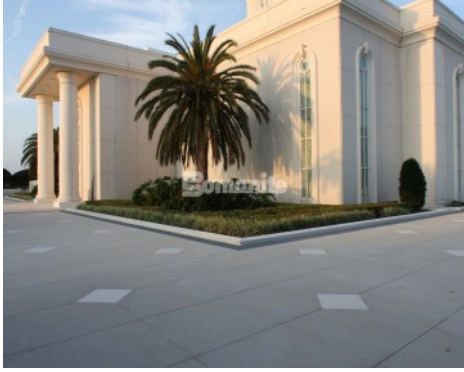
Church of Jesus Christ of Latter Day Saints in Windermere, FL, Exposed Aggregate installed by Edwards Concrete Bomanite.
