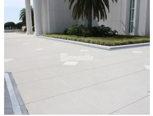
Church of Jesus Christ of Latter Day Saints in Windermere, FL, Exposed Aggregate installed by Edwards Concrete Bomanite.
