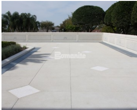
Church of Jesus Christ of Latter Day Saints in Windermere, FL, Exposed Aggregate installed by Edwards Concrete Bomanite.
