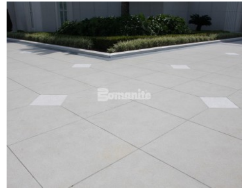
Church of Jesus Christ of Latter Day Saints in Windermere, FL, Exposed Aggregate installed by Edwards Concrete Bomanite.
