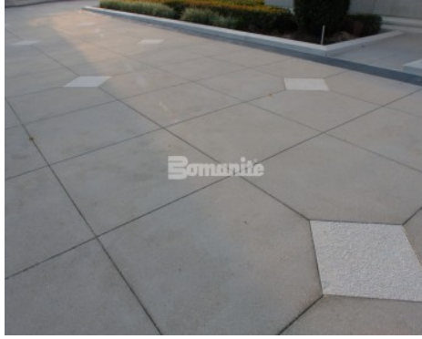
Church of Jesus Christ of Latter Day Saints in Windermere, FL, Exposed Aggregate installed by Edwards Concrete Bomanite.
