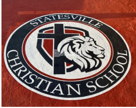
Statesville Christian School in NC featuring Micro-Top XT installed by Carolina Bomanite Corporation.
