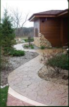
▶ ...you can improve resistance to Deicing Chemicals with the correct installation of imprinted concrete? By using a Bomanite Contractor they will ensure that Bomanite Color Hardener is used if possible, the surface of the concrete will be sealed and the use of Bomanite Con-Shield as a pre-treatment prior to sealing will be used where Color Hardener was not utilized.
