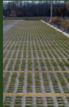
▶ ...that Grasscrete is ideal for sustained traffic areas and can be partially concealed with vegetation so it is functional, environmentally friendly and pleasing in appearance? Shrubs or trees form a softer, natural marker than do curbs or bollards and can be easily incorporated into most trafficked applications as delineation for vehicles. With its self-draining nature, Grasscrete can be cast to within 24" of mature trees. To learn more about Grasscrete, [Click Here](#).
