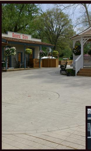
The Bomacron Circular Granite Stone can be installed at a 2 1/2' radius and up to a 10' radius. Individual stone sizes average 5" square.
