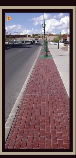
The Bomacron Running Bond Used Brick Pattern uses a a traditional recycled brick texture set in a pattern replicating hand laid brick paving. Containing moderate to light depth of relief and intended for use anywhere that typical brick or masonry unit paving is desired, individual brick sizes are available in 4" x 8" as well as 2 1/4" x 7 1/2".
