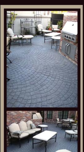
The Bomacron Fishscale Granite Radius pattern has a uniform texture of moderate depths of relief consistent with cleft granite stone.
